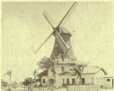
DE OLDE MOLEN , here is truly a little bit of Holland in the Caribbean. An authentic 150 year old windmill, shipped disassembled from Holland and reconstructed a breeze away from Aruba's "côte turquoise" hotel strip. The old "windmill" houses a fine restaurant, bar and swinging nightery.
